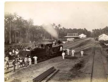
Construction of Matara railway line in 1895
